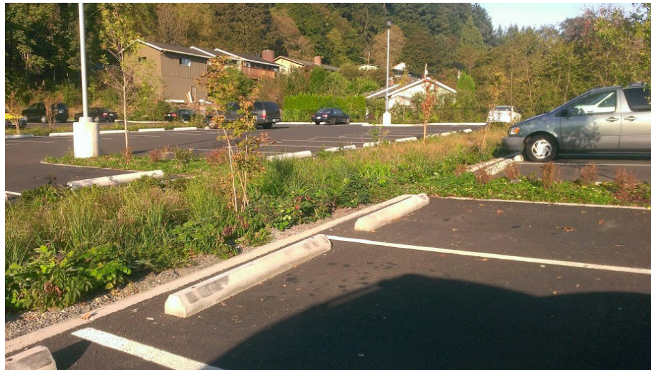
VEGETATED STORMWATER BASIN IN PARKING MEDIAN
