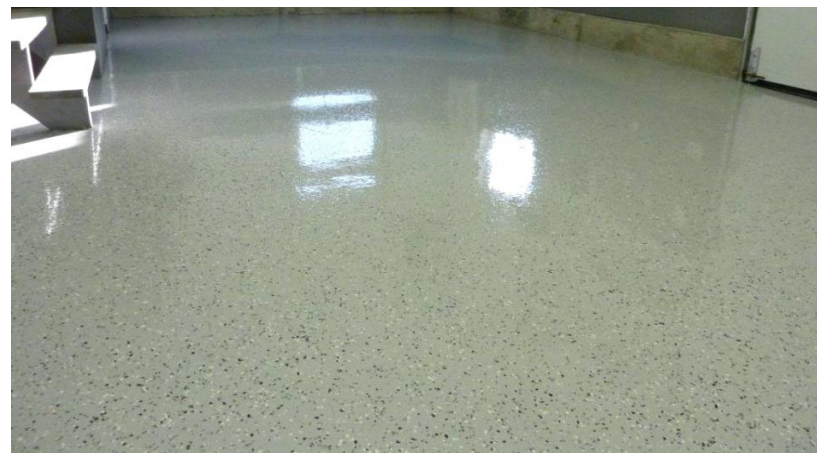
POURED EPOXY FLOORING
