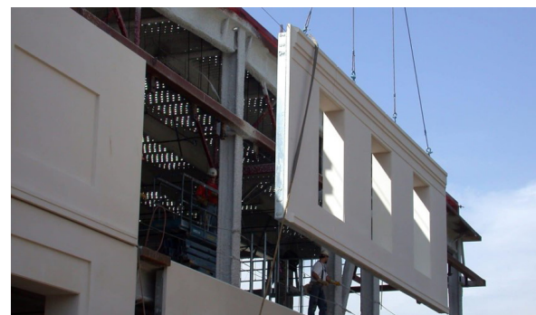
CONCRETE TILT, PRECAST CONCRETE, AND RAINSCREEN CLADDING WILL BE USED STRATEGICALLY ON THE KELLOGG BUILDING ENVELOPE
