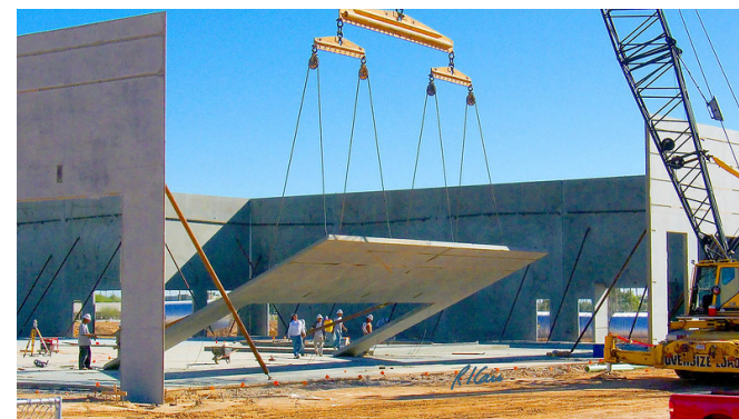
TILT UP CONCRETE WALL LIFTING
