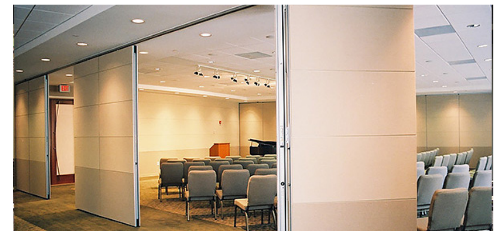
EXAMPLE OF OPERABLE FOLDING PARTITIONS WITH ACOUSTIC TREATMENT FOR STAGE
