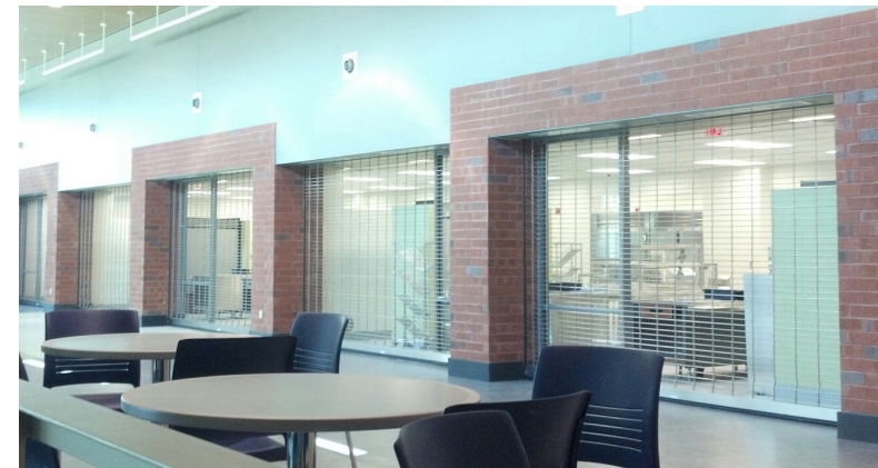
COILING DOORS WILL BE USED TO LOCK OFF THE SERVERY AFTER HOURS
